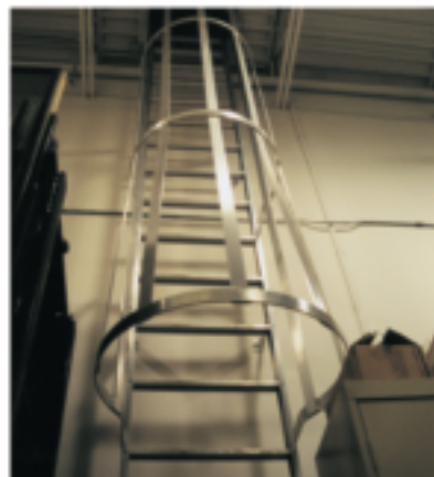
Fixed Aluminum Wall Ladders
